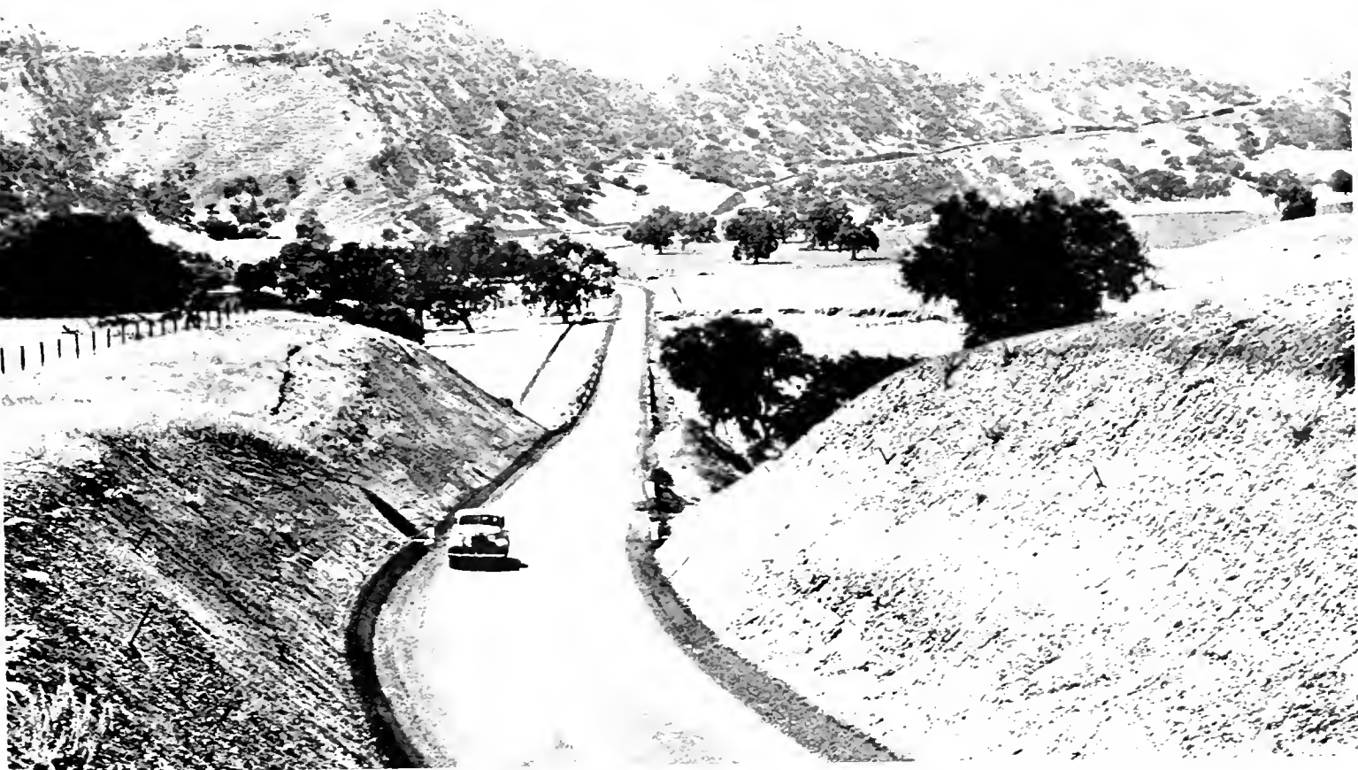
Two views of improved sections of realigned Mustang Ridge route through mountains separating San Joaquin and Salinas Valleys where a narrow old road with 123 sharp curves in 5.3 miles has been replaced by a 21 foot highway with 23 easy curves.
